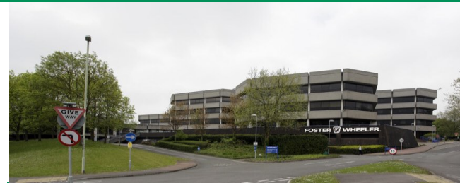
Shire Hall, Shinfield Park, Reading
