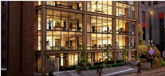
28 Dingwall Road, Croydon
